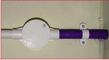
Fireblok® conduit sleeve fitted into a 20mm BESA box
