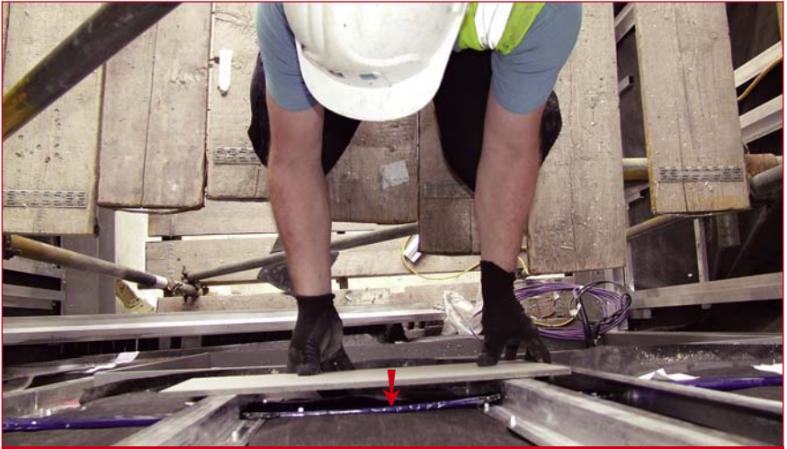
FIRE BARRIER PROTECTS GAP BETWEEN WALL AND CLADDING
