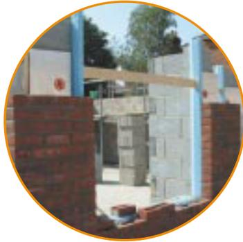
3 Can be used in conjunction with all types of cavity wall insulation. Thermabate's wall fixing ties are used to secure the profile in position.
