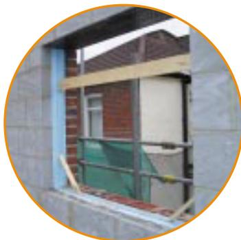
The closer sections are delivered pre-formed, assembled into a frame to specified sizes around which the wall is built, for the window frame to be installed later.
