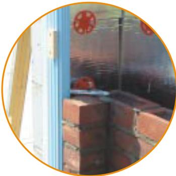
4 An insulated lintel or Thermabate can be used at the head. Plastic, timber or metal window frames can be used with Thermabate<sup>2</sup>, fixed independently to either leaf of construction.
