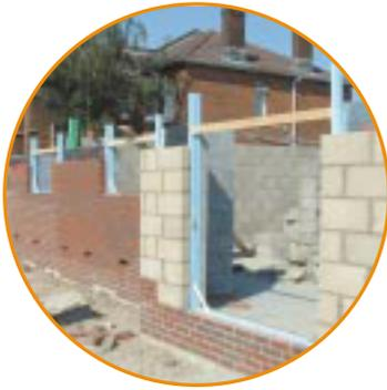
1 Available in cavity widths 50mm, 65mm, 75mm, 85mm, 90mm & 100mm. A tolerance of up to 10mm can be taken up behind the fixing flange to give a range of widths from 50mm to 110mm.
