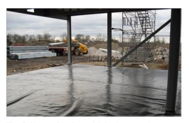
If installed incorrectly or damaged during the construction process, the membrane is rendered ineffective and will fail to provide adequate protection against the ingress of ground gas or vapours.
